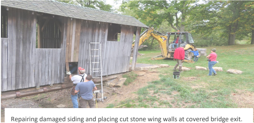
Repairing damaged siding and placing cut stone wing walls at covered bridge exit.
